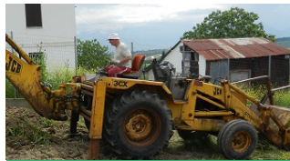
JCB Clearing Area
