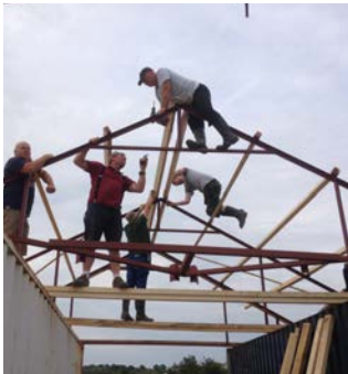
Men working on the roof
