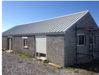
Camp In Progress
